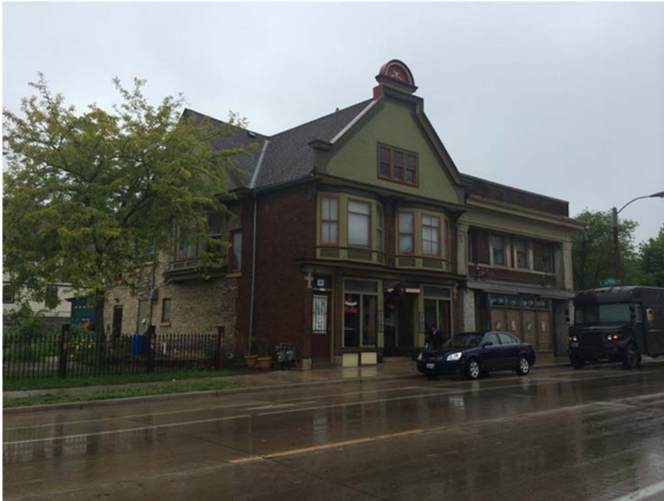
Street view and façade.
