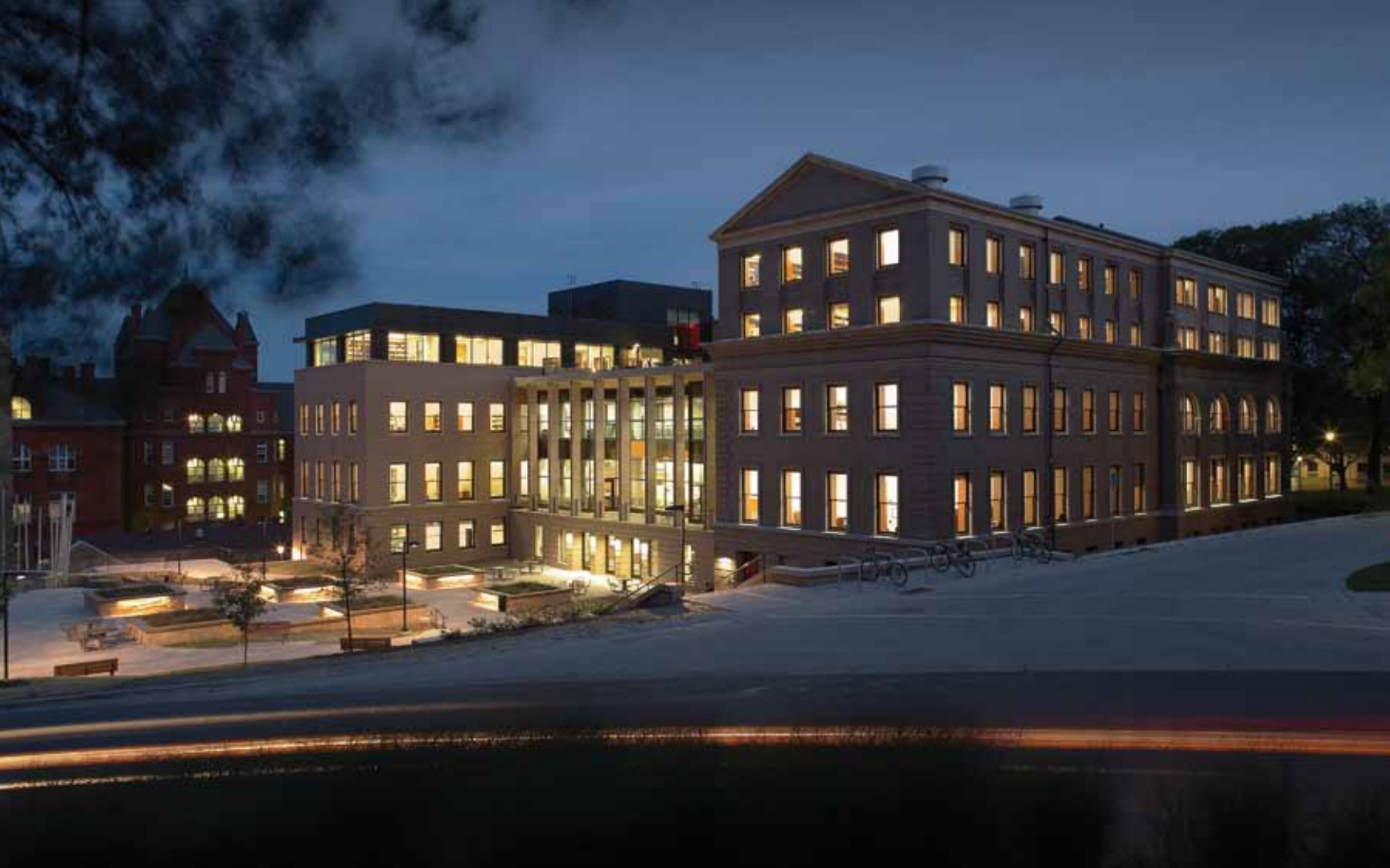
The School of Education with a green roof plaza over parking (at left), the new east wing, the central atrium, and the 1910 west wing (at right).
