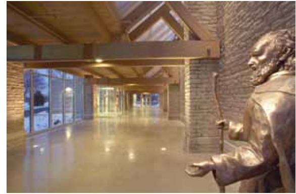
The new timber-framed and sky lit narthex at St. Anthony's, with the 1854 stone façade at right.
