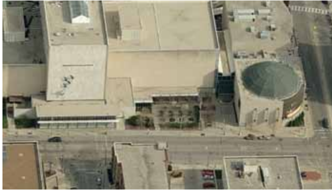
The linear Vivarium at left, the new entry courtyard, and the 1994 IMAX Theater (at right).
