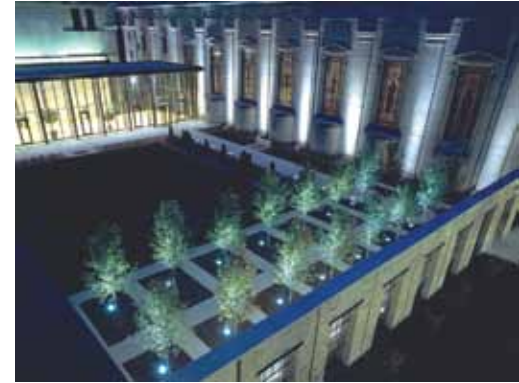
View of the new garden courtyard with the glass loggia at left.
