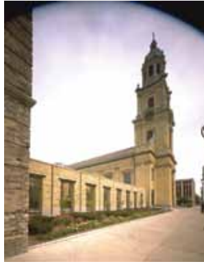
The "After" view with the new courtyard.
