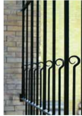
A detail of the garden wall ironwork.
