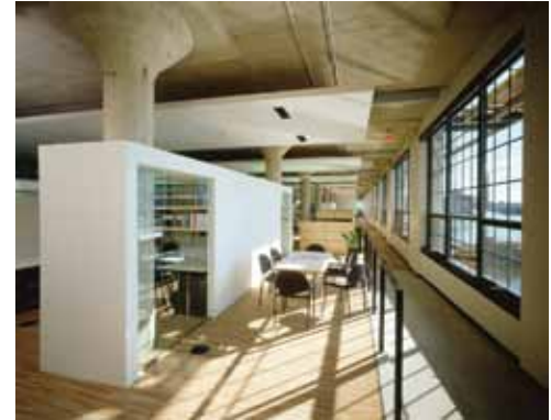
In the office spaces, board-formed concrete structure is exposed.
