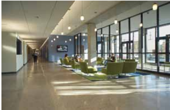
Floors in the commons were made of polished concrete embedded with glass.
