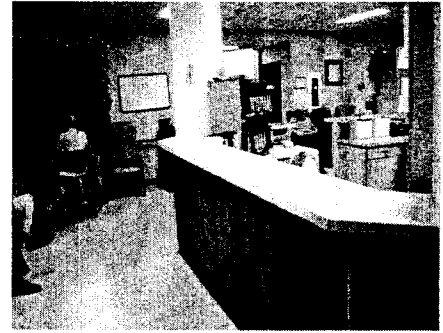
Pre-renovation: Dominant physical presence of the nurses' station at the crossroads of hallways made a strong institutional statement.
