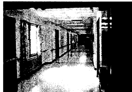
Kingswood Health Center: Pre-renovation view of long double-loaded hallways with institutional finishes
