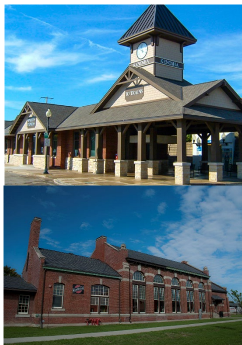
Figure 1 – Existing C&NW Stations in Kenosha (top) & Racine (bottom) to be utilized
