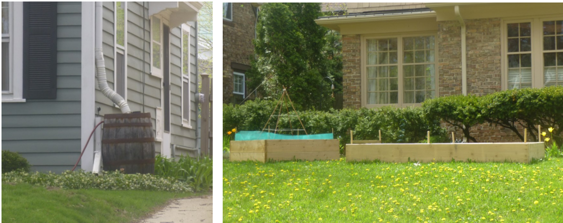
From Left to Right: Downspout Disconnection and Rain Garden in Shorewood
