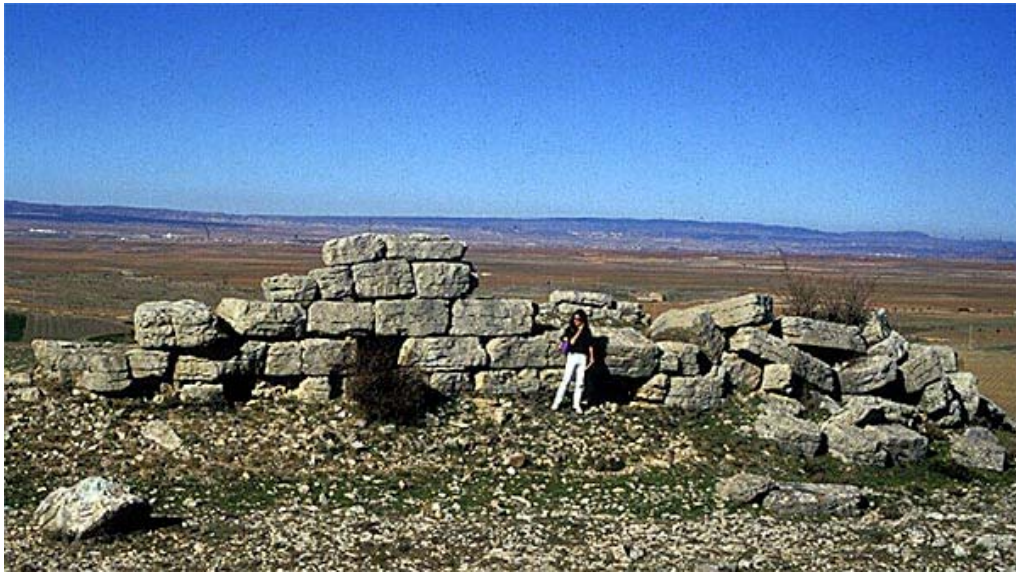
Figure 14. Small fortifications of Sierra Menera, Teruel (photo F. Burillo).
