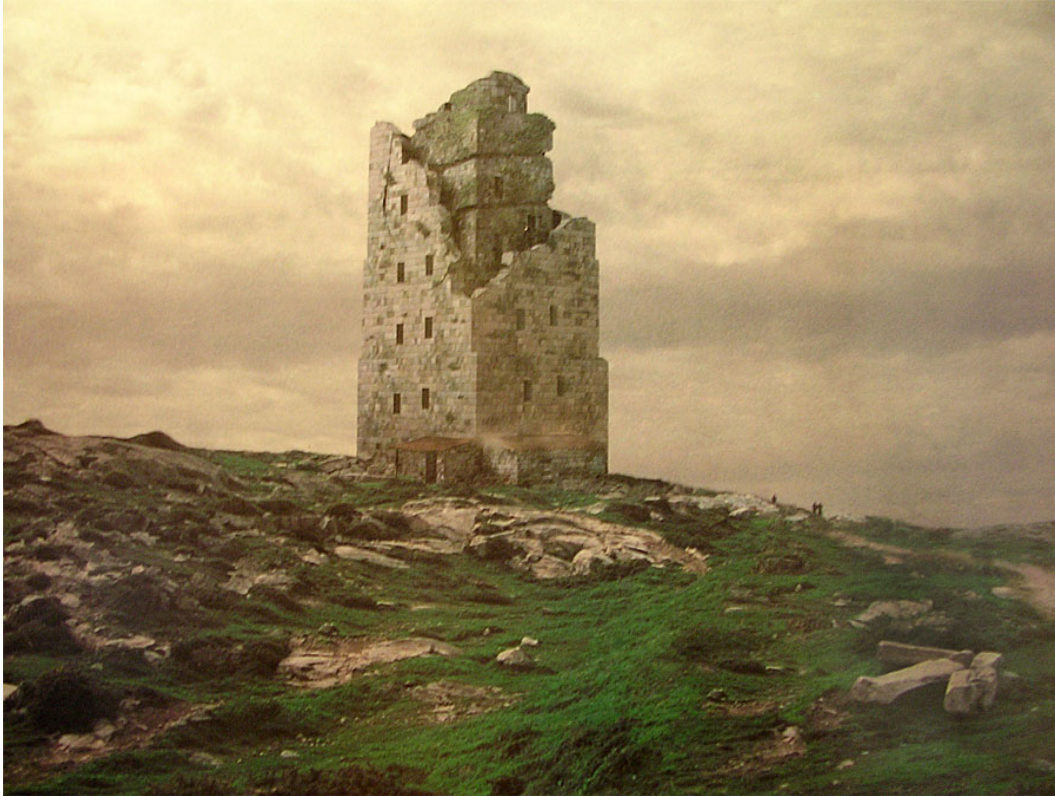
Figure 1. Here we have one of the earliest images of the Torre de Hércules (the Tower of Hercules). It was constructed by the Romans in the second century BC (Photo: Alfredo Erias).
