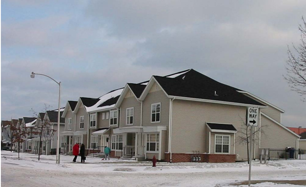
Figure 9: New Covenant Housing, Milwaukee 2005
