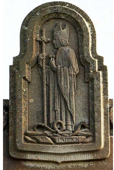
Figure 9. Exterior molding, Jurby Church.
