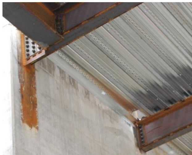
b) rigid girder-wall connection
