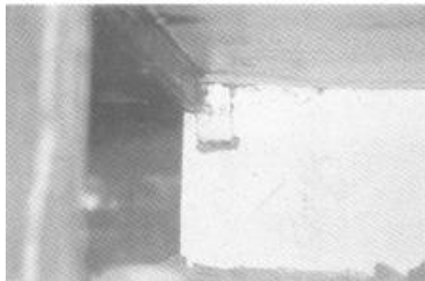
Fig. 2.3 Girder-wall connection failure in the model structure by Li et al. (2002)
