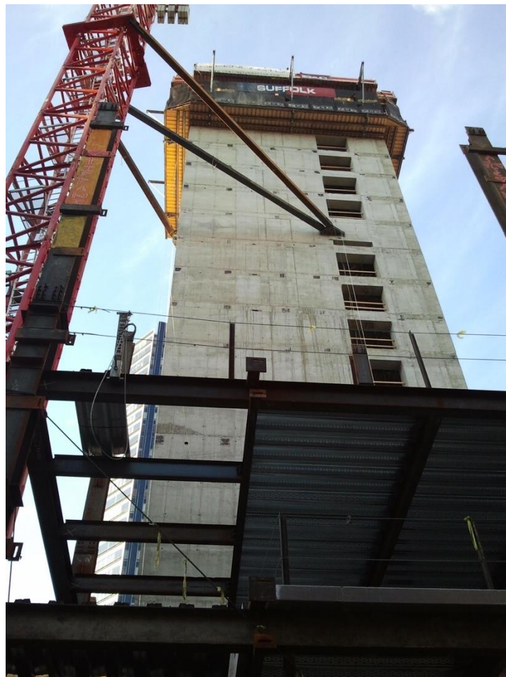
Fig. 1.1 Composite construction for high-rise building structures
