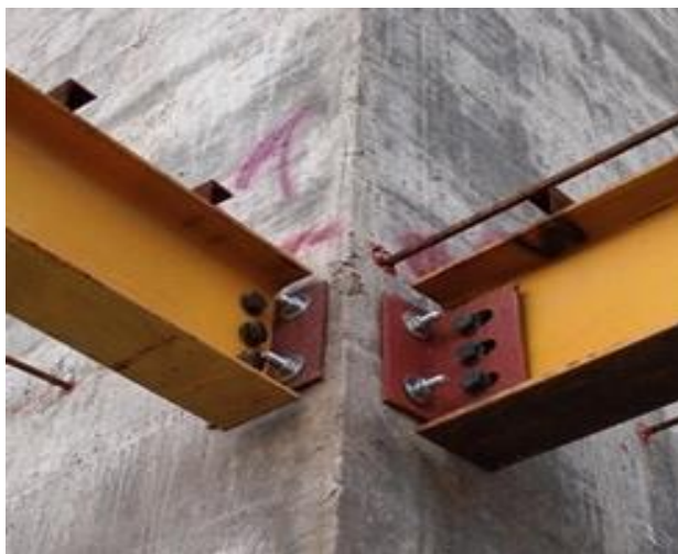
a) pinned girder-wall connection;
