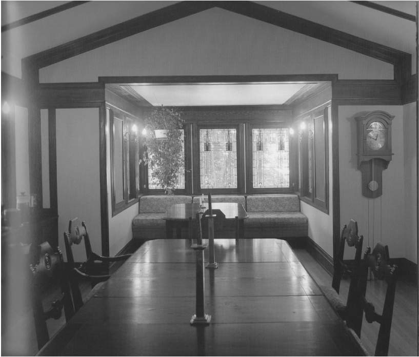
Thomas Residence, 1901: Notice corner trim at wall corners and upper soffit:
