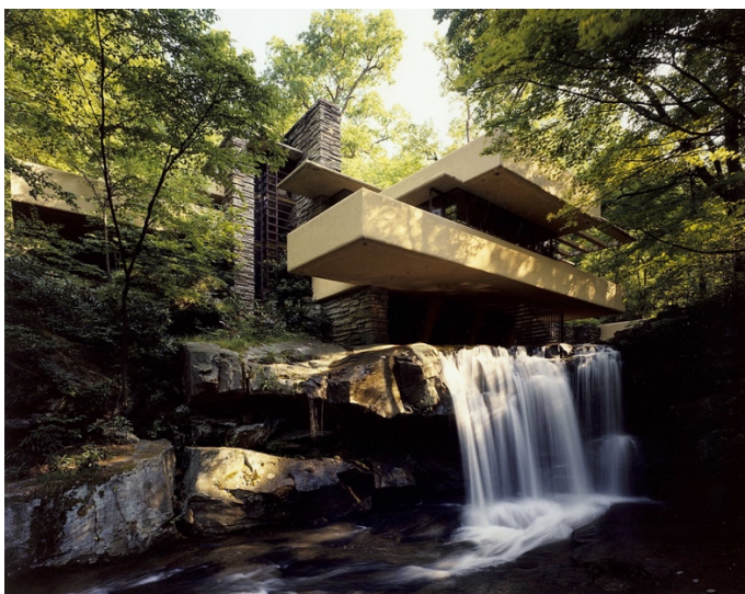
Figure 3.31. Frank Lloyd Wright, Fallingwater, 1937.
