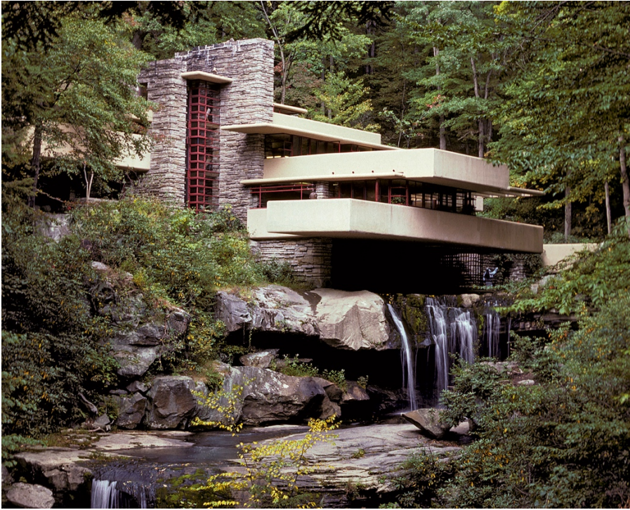
Figure 4.6. Frank Lloyd Wright, Fallingwater exterior. 1937.
