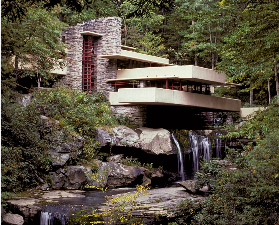
Figure 2.1 Frank Lloyd Wright, Fallingwater. 1937.
