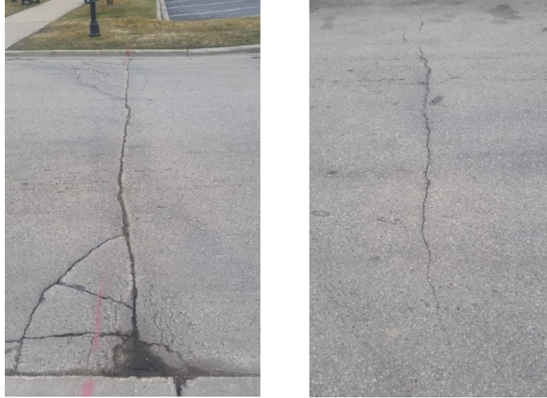
Figure 2.14: Low-Temperature Thermal Cracking
