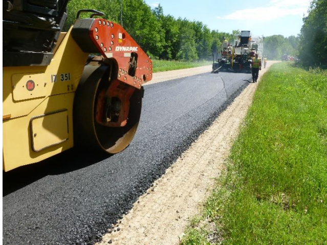
Figure 6.1: Wausau, WI Road Paving Project
