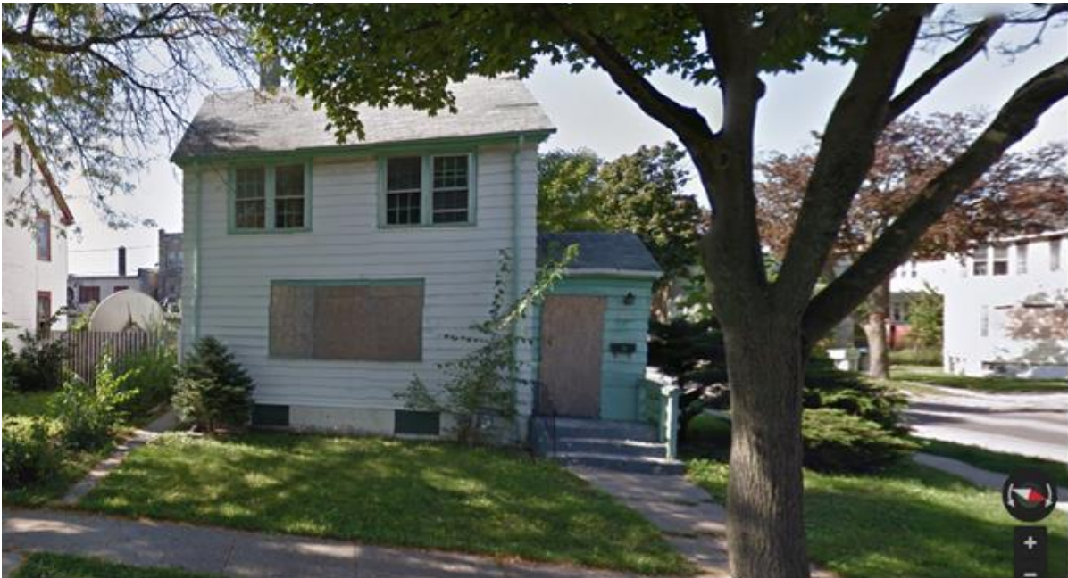
Figure 3-2 - Garden Homes District – Now
