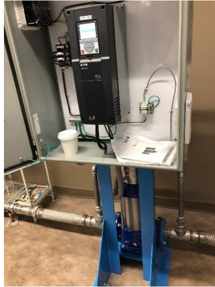
Figure 14- Pump's safe mode controller
