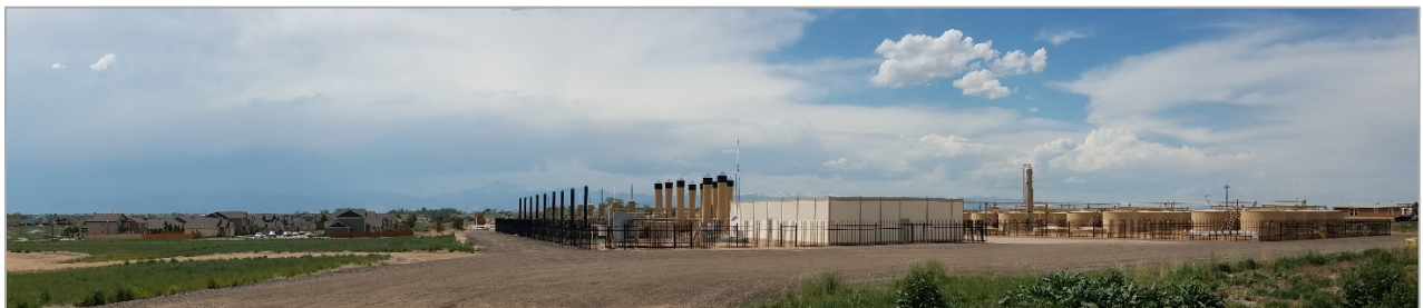
Figure 3. Large multi-well oil and gas production facility near residential subdivisions in the Town of Mead in Weld County, Colorado (Photo by the author)
