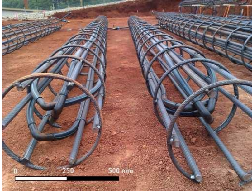
Figure 1-8- Reinforcement cages with the attached fluid-carrying pipes.
