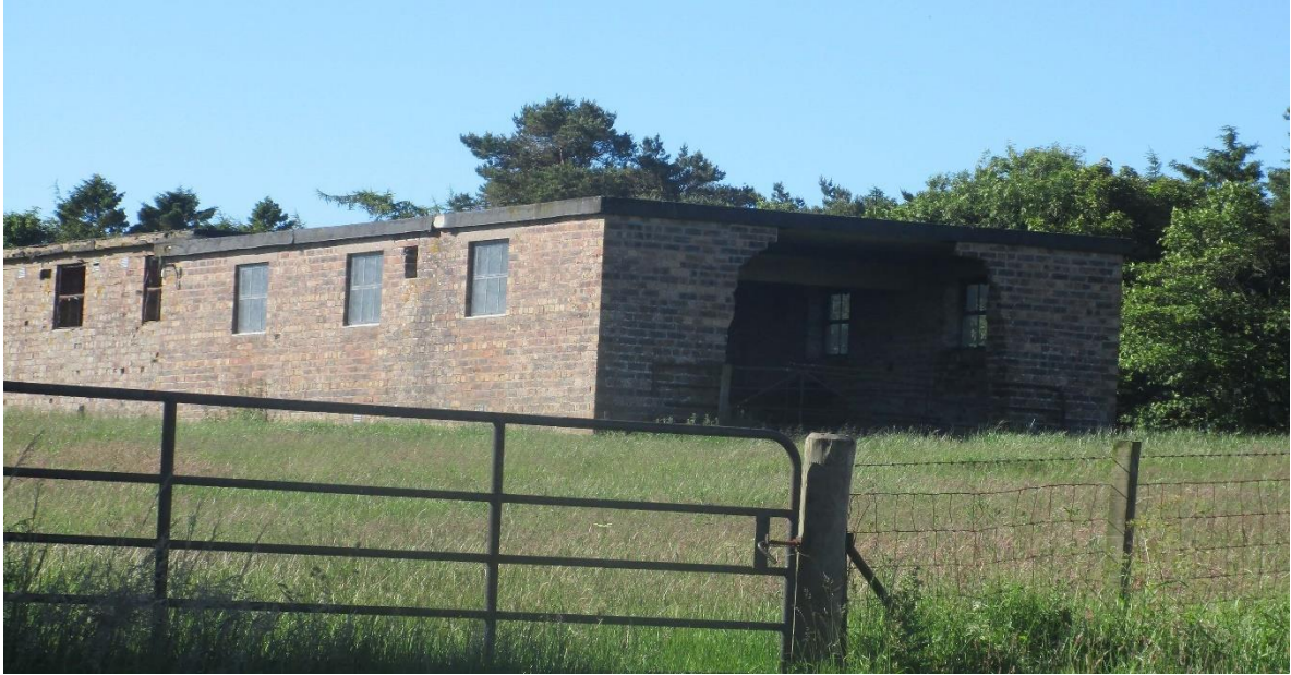
Figure 3. 1: Abandoned building on road leading to the FallOut Bunker.
