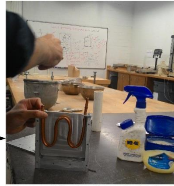
Assemble the inserted tube in the concrete mold
