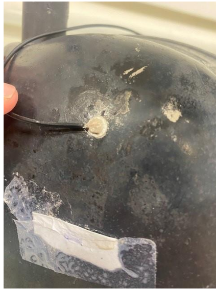
Figure 3.4: Close up view of PZT mounted on tank.
